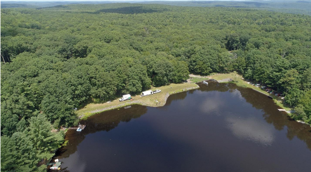
Dive team preparing to inspect the Walker Lake dam.
