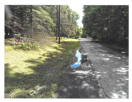
Notice the width of the roadway in the background of where the puddle is ... look at the deterioration the water is causing at this location also causes premature failure of road area next to it (see the extensive cracking)
